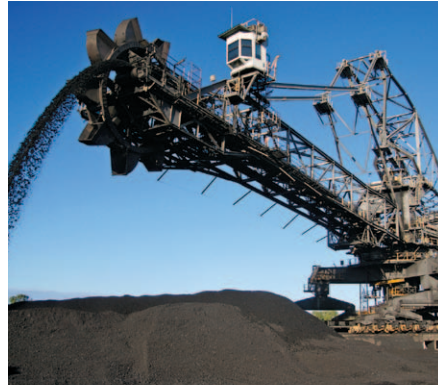
Coal stacker and reclaimer
